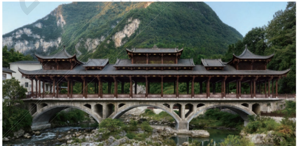
Feiyue Fengyu Bridge and Feiyue Cattle Shed by RLX Technology
