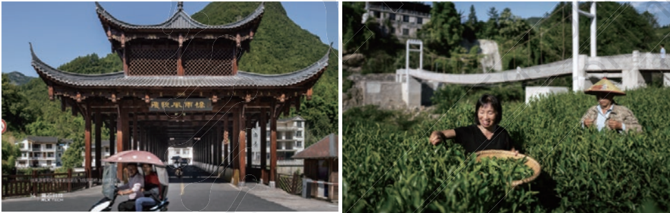
"Feiyue Fengyu Bridge" and "Feiyue Convenience Bridge," Source: RLX Technology Official Website
